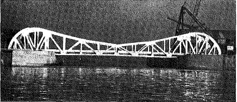
Fig. 1-3. The twin bascule bridge at Hendon Junction, Sunderland, Co. Durham – the world's first all-aluminium structure of this type
