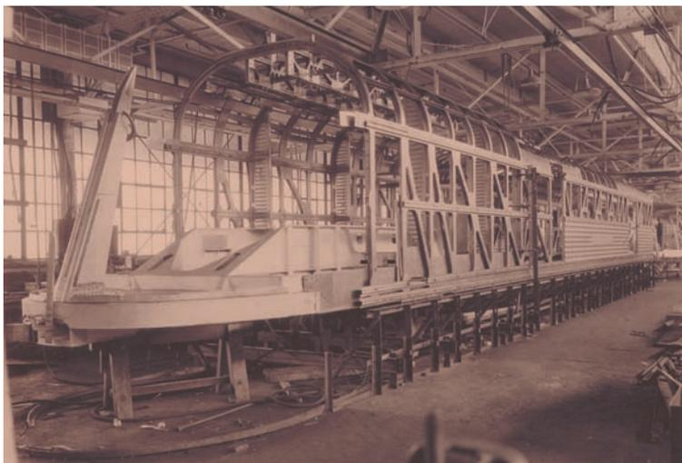
The front car of the Burlington Zephyr under construction. Note the two stanchions that support the diesel engine at the front of the car. (Hagley photo)
